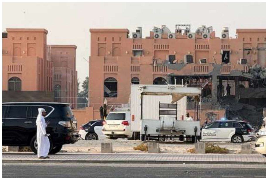
A damaged building, following an Israeli attack on Hamas leaders, in Doha, on September 9. REUTERS
