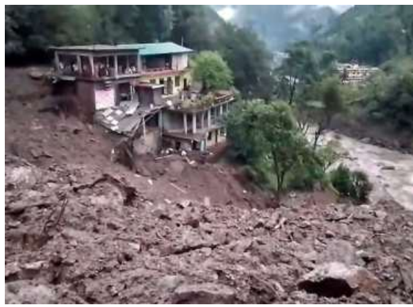
Down to rubble: Several houses lie damaged due to landslides in Nandanagar area of Chamoli district, Uttarakhand on Thursday. PTI
